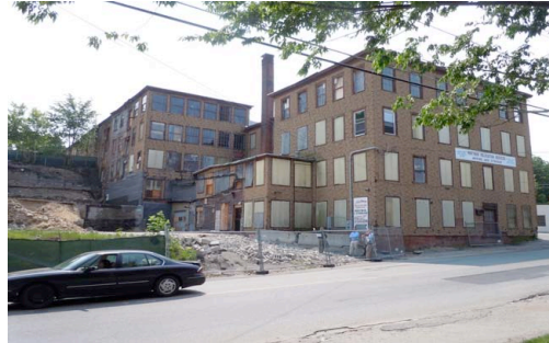
Whitney Building, pre-construction
