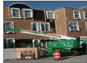
Turtle Creek, Beverly: Construction underway
