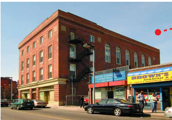
Hibernian Hall, a formerly vacant historic building now used for social and cultural events, youth activities, and job training
