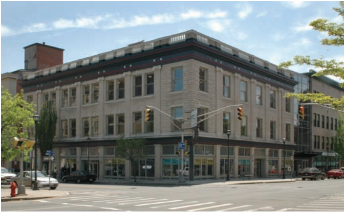
Holyoke Health Center, Holyoke, Massachusetts MHIC provided NMTC allocation and syndicated the tax credits
